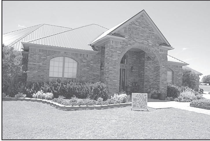
WARD ONE —1155 Old Caufield Road, Prince Anderson
