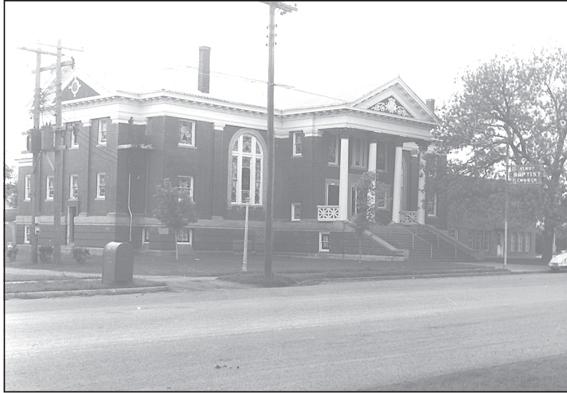
First Baptist Church Greek Revival Sanctuary was built in 1913.
